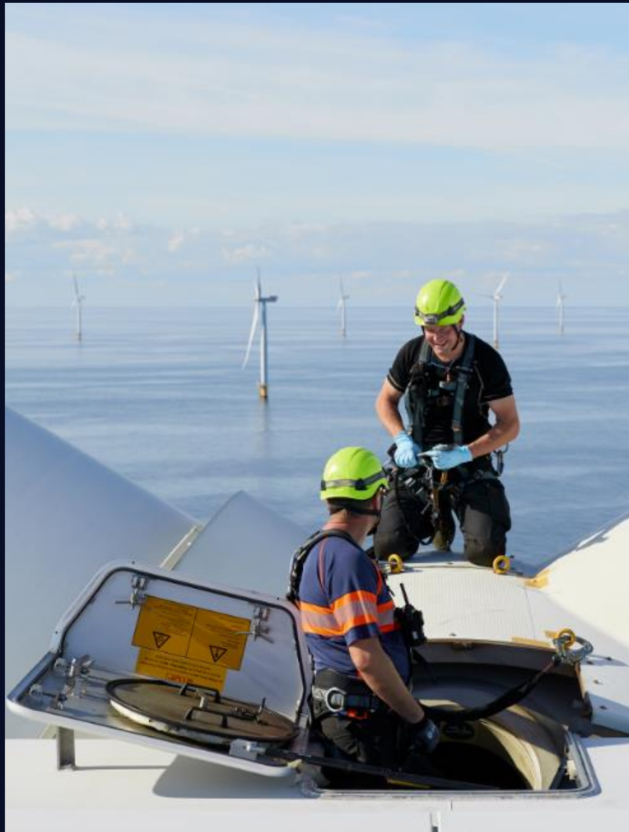
Anholt wind technicians, Courtesy: Orsted
